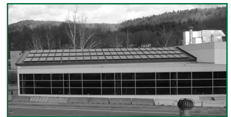
Southern Vermont Recreation Center's existing solar thermal system at work.
